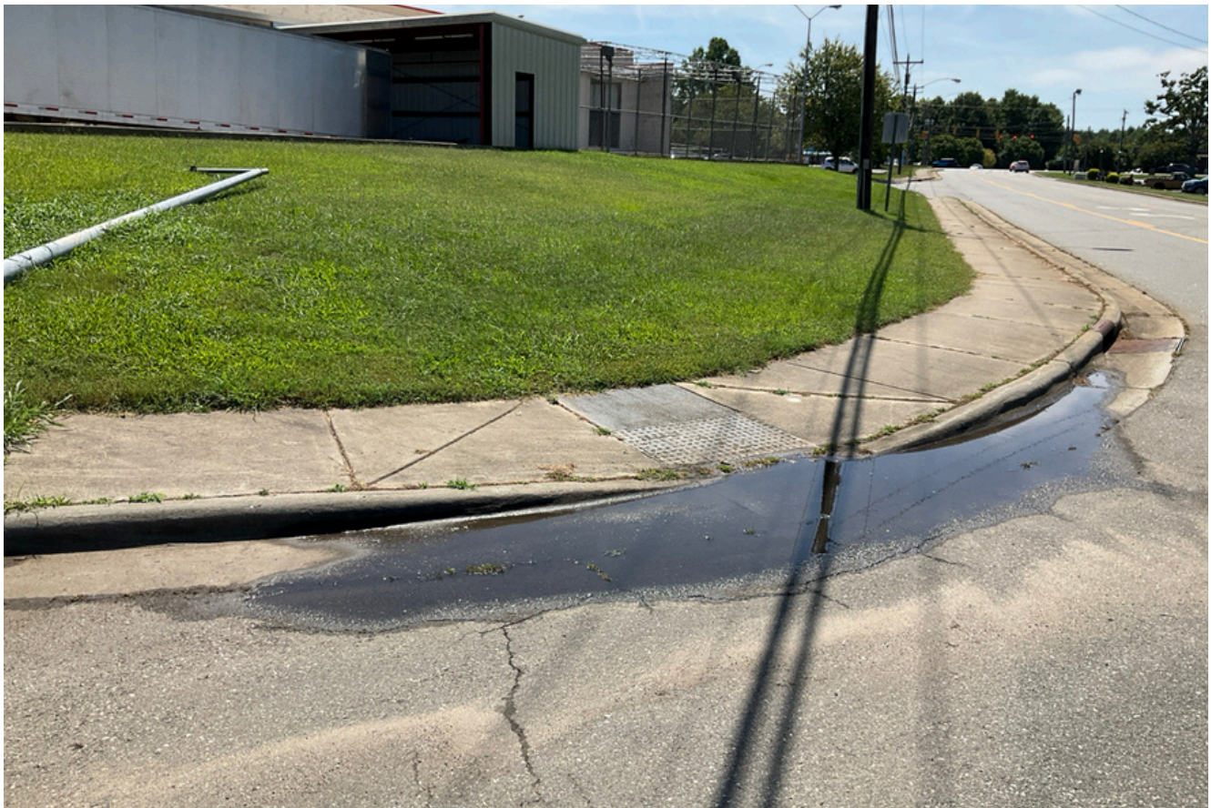
Caption: Curb ramp with ponding.
