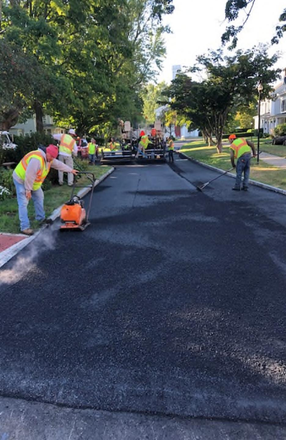
A photograph showing a group of construction workers in safety vests and hard hats working on a paved road. One worker in the foreground is operating a small orange vibratory plate compactor. Other workers are visible in the background, some with shovels and a wheelbarrow. The road is dark asphalt, and there are trees and houses in the background.
